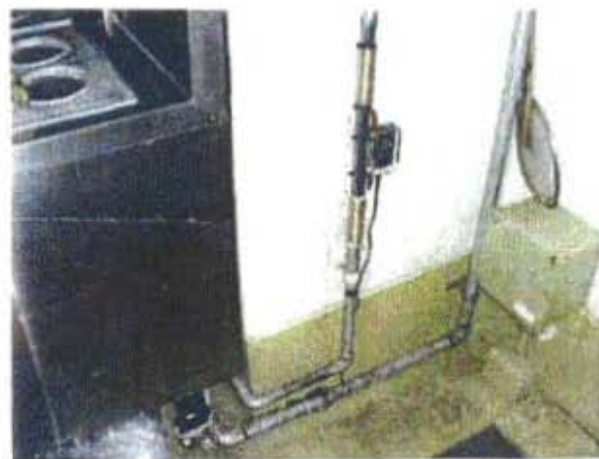
Water treatment system installed
