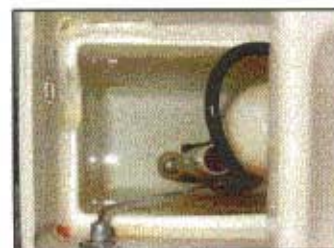
[Cleaned with sponge thirty minutes after the installation of the Vulcan]
