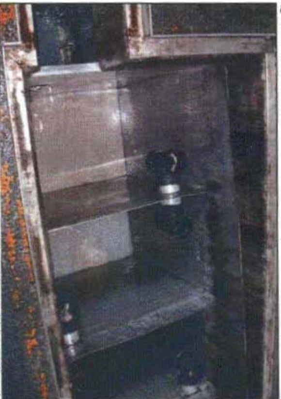
The first tank: Upon high pressure cleaning (grease is adhered on the inside walls)
