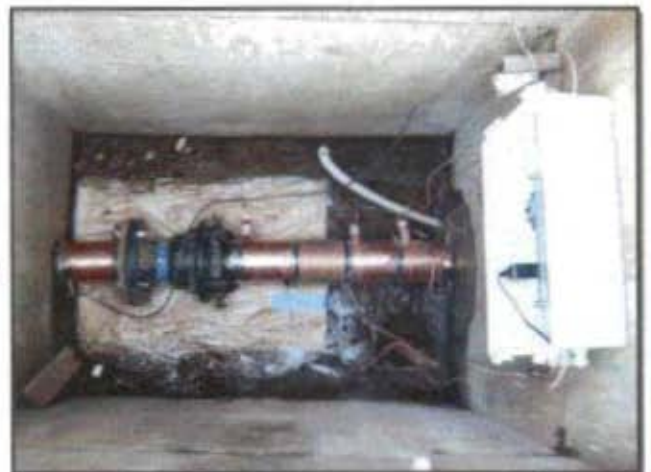
[Cable winding completed]
