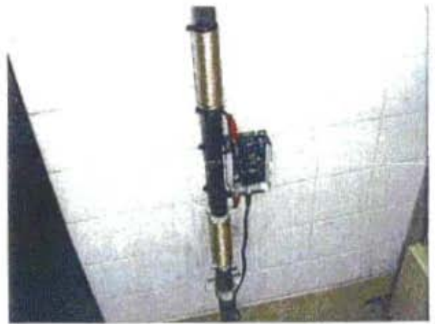
Main body of the water treatment system installed
