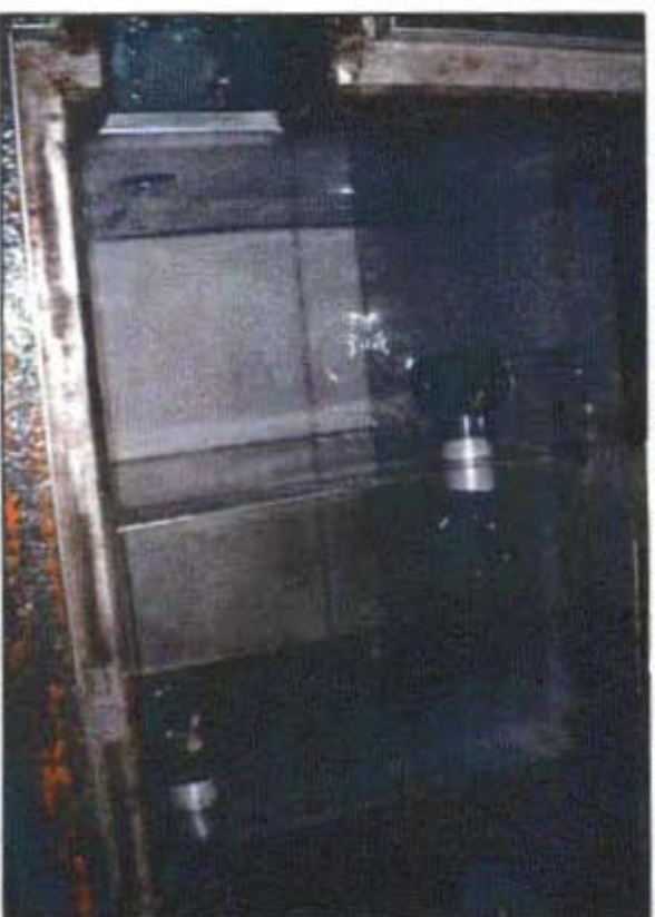
The first and the second tanks: Upon cleaning by rubbing using detergent
