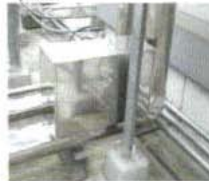
Used for the cooling towers A, B, and C
