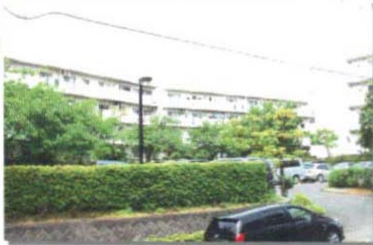
[Overall view of the apartment building]
