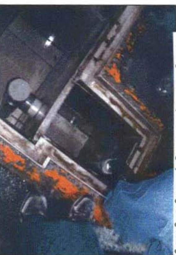
Drainage tank: Upon cleaning by rubbing using detergent
