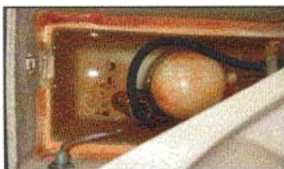
[Before installation of the Vulcan]
