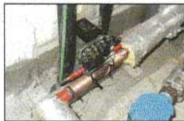
[Installation of the Vulcan completed]
