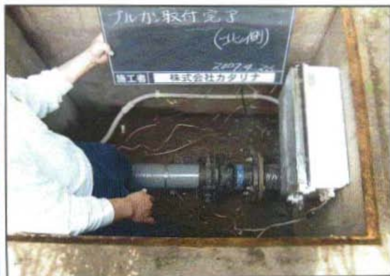
[Installation of the Vulcan completed]
