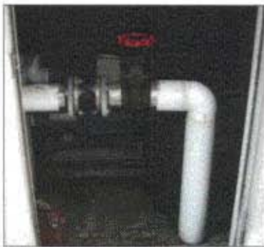
[Before installation of the Vulcan]
