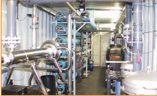
Sea water desalination 500 m 3 /day
