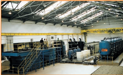
Water works 5.000 m 3 /day
