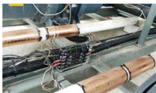
Vulcan S100 was installed on the main air-conditioning system
