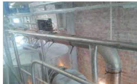
Installation of Vulcan S100 on lime kiln
