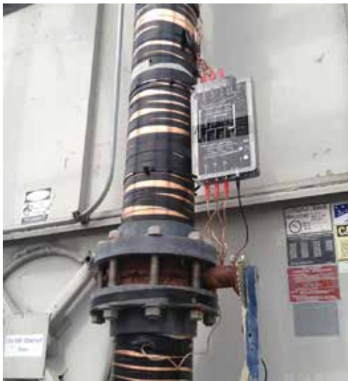
Vulcan S100 installed on cooling towers
