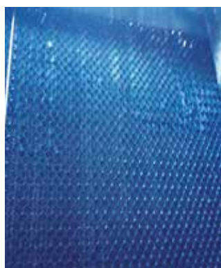
This photo was taken of the inside of CT-1.
