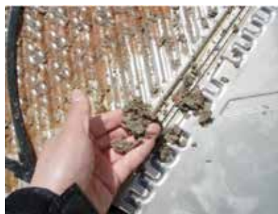
The scale can be easily removed.
