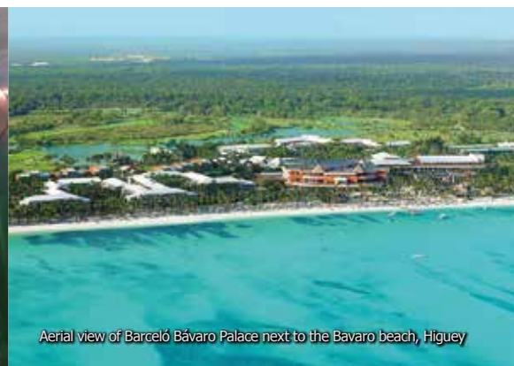
3 chillers were treated by 3 Vulcan S500
