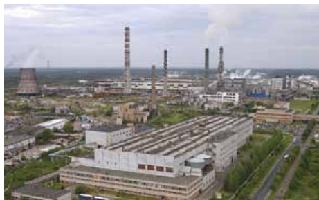
Mondi Štětí a.s manufacturing plant in the Czech Republic
