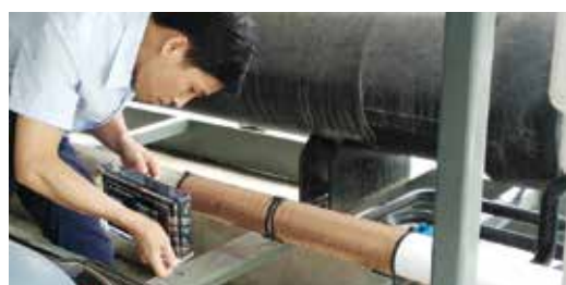
Installing Vulcan S100
