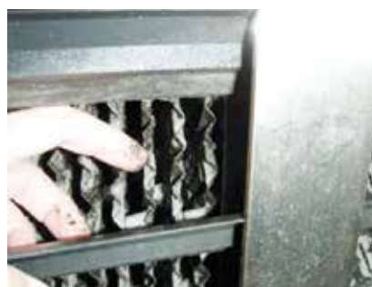
After Vulcan was installed for 5 months: the scale can be removed easily with a finger.
