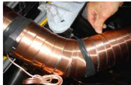
Vulcan Impulse Cables double wrapped on water pipe
