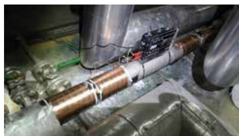
Vulcan S25 installed at Toray Industries
