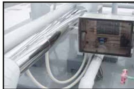
Impulse cables and the Vulcan S25
