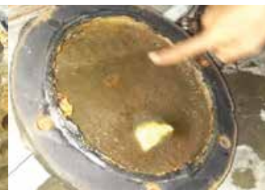
Inside of heat exchanger. Condenser end plate had lost all scale that was there previously. (Light spot at bottom is reflected light.)
