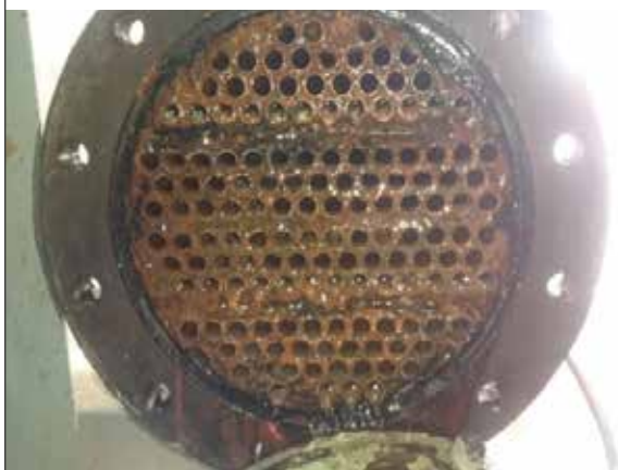
Heat exchanger before Vulcan installation
