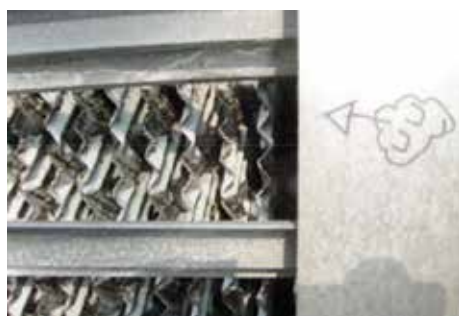
Before Vulcan was installed: the outside of the cooling tower.
