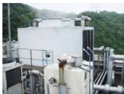
The cooling tower roof of medicine factory
