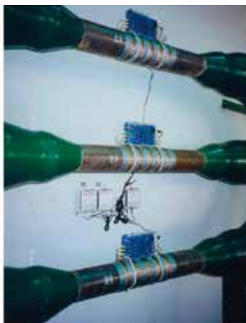
After Vulcan installation
