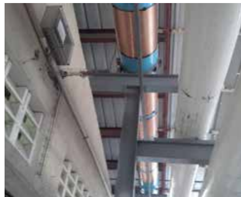
Vulcan S500 cable windings
