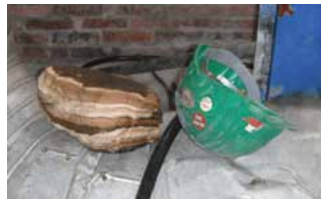
Deposit removed from pipe after Vulcan installation
